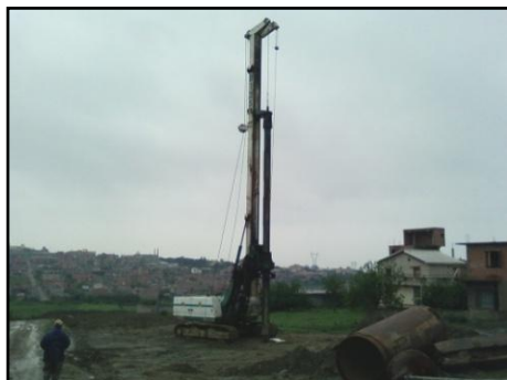
Figure C.3. Fraise hydraulique de forage
