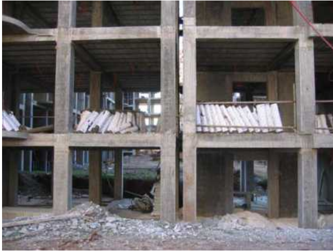
Figure 5.29 c). Joint sismique.
